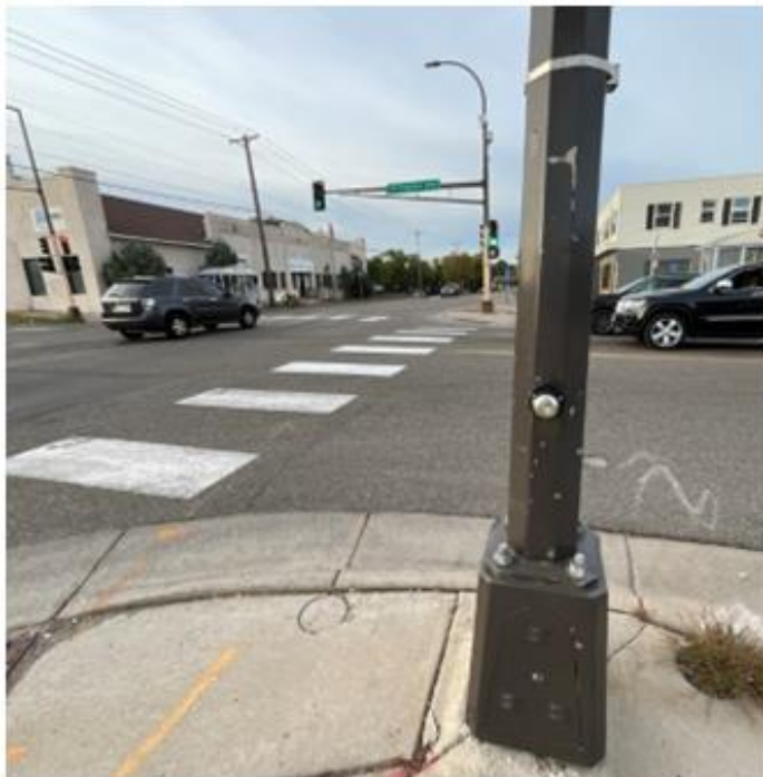
Non-Compliant Push Button
