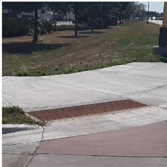
Compliant Curb Ramp With Truncated Domes
