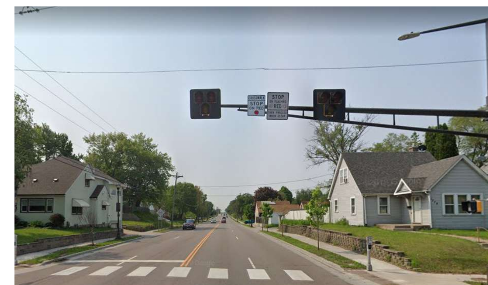
Pedestrian Crossing Signals
