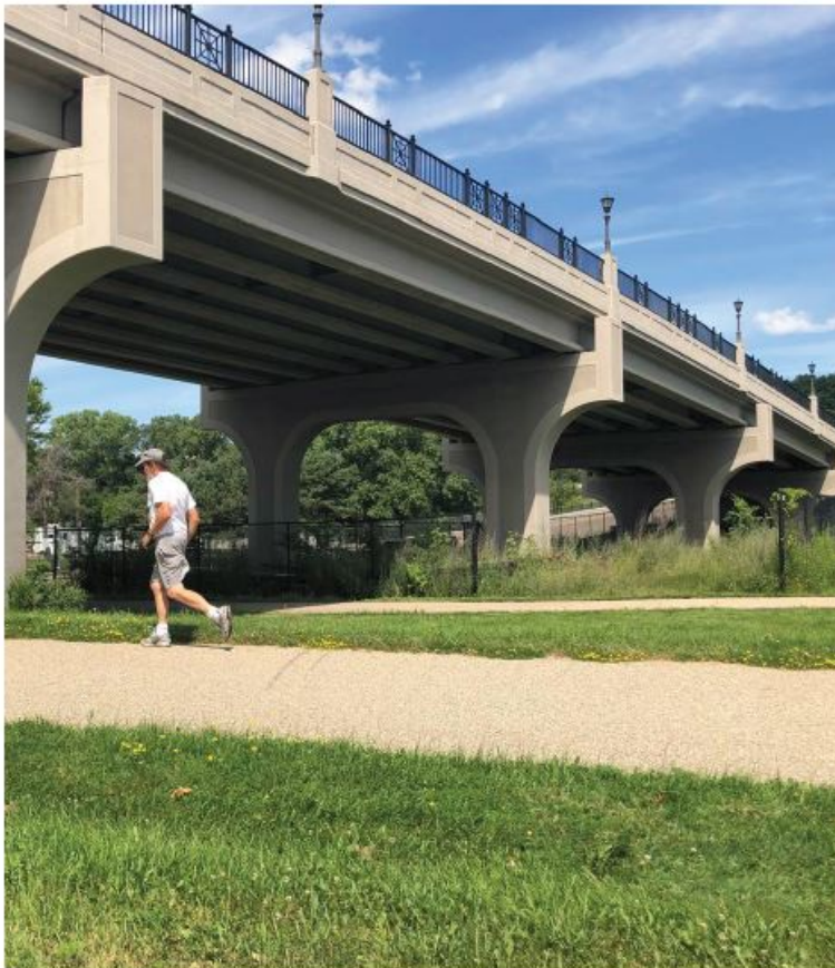
EXISTING EARL STREET BRIDGE
