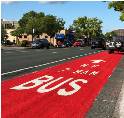
City of Minneapolis Installation of Red Marking Treatment
