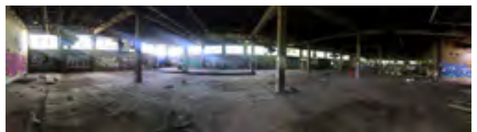
Interior View of Building 189 Point 1, Page 3
