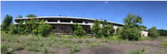
Exterior View of Building 189
